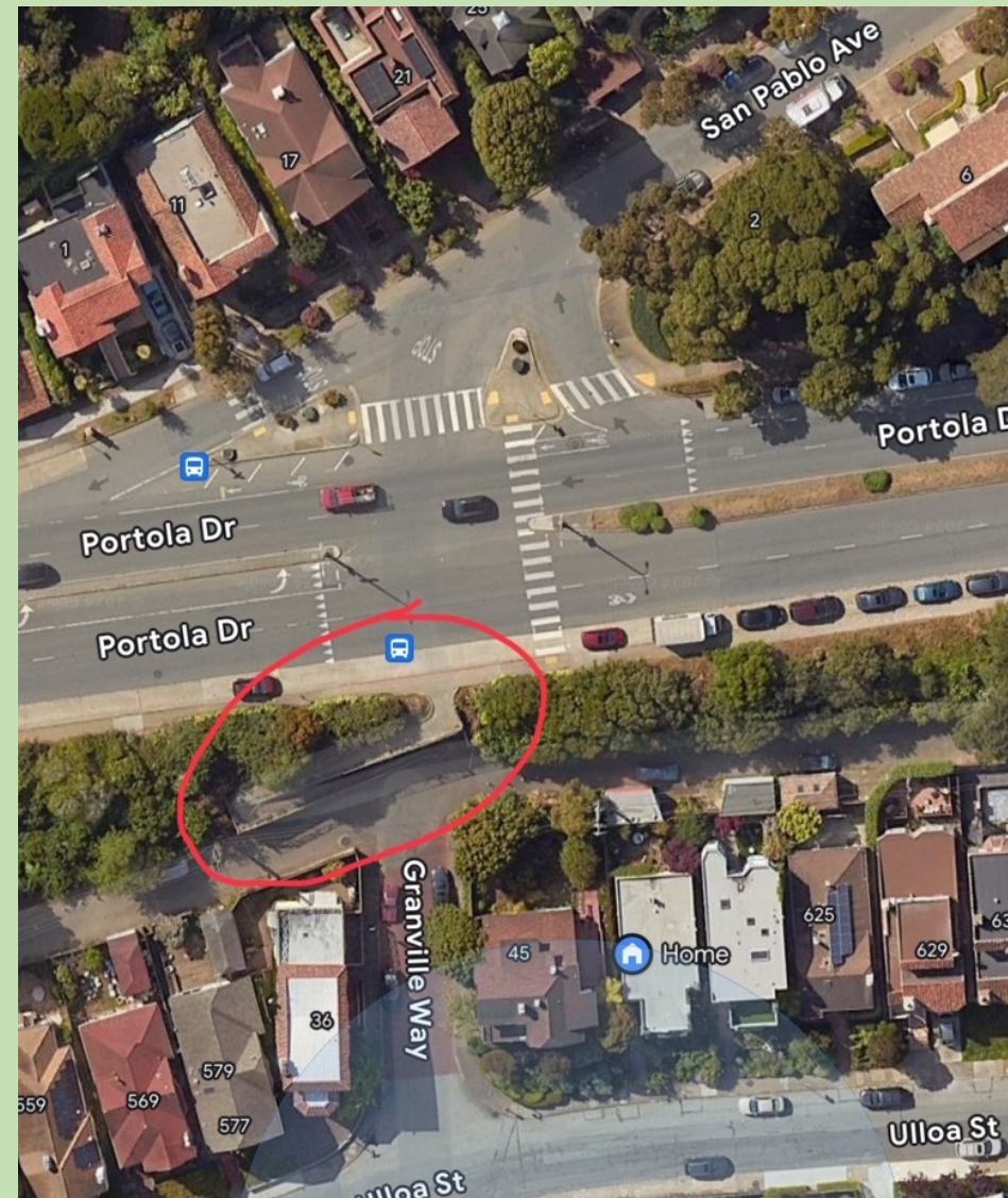
Pedestrian ramp connecting Ulloa with Portola
