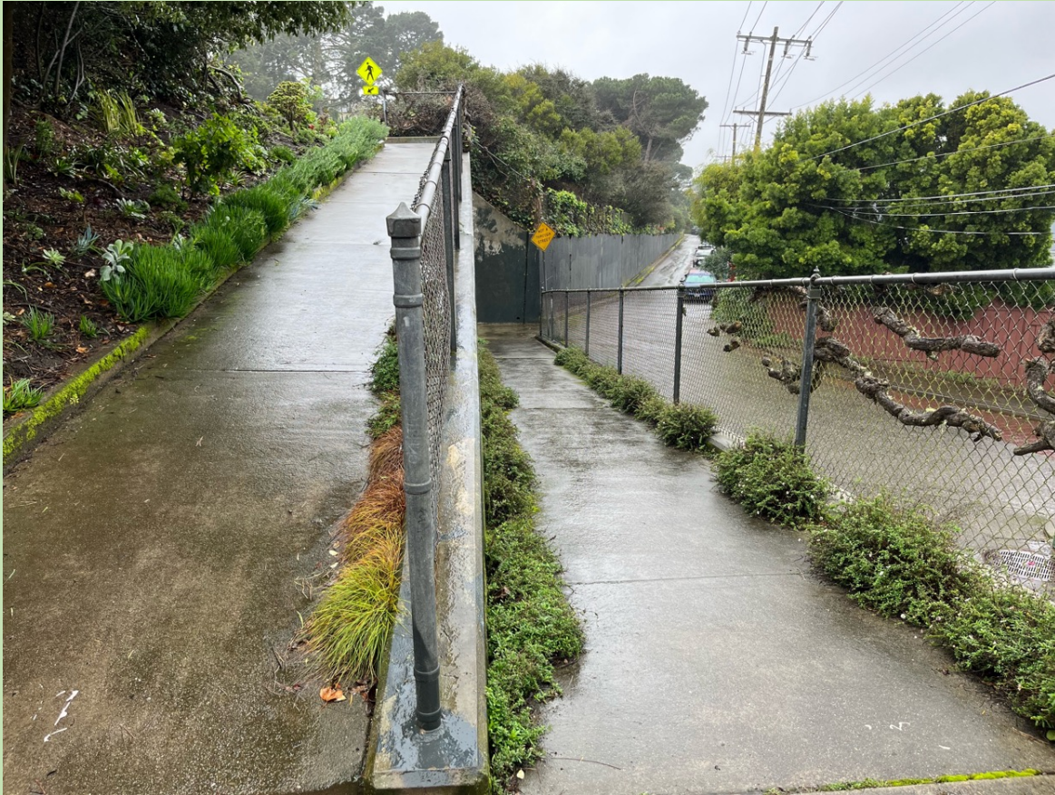
The Ramp, notice the ivy stumps intertwined in the cyclone fence.
